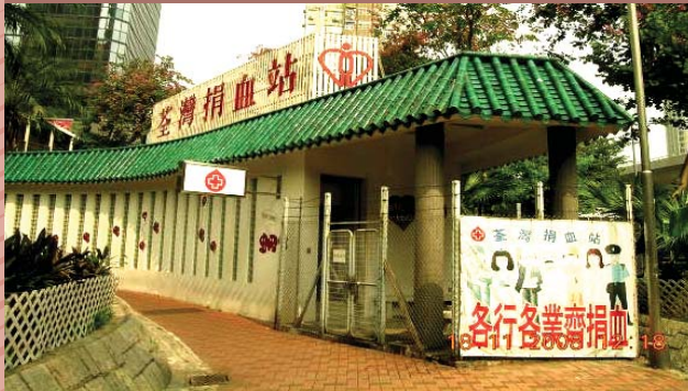
舊貌 Before Renovation
